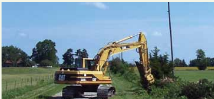
2 The trackhoe removes all trees and vegetation without damaging existing fences.
